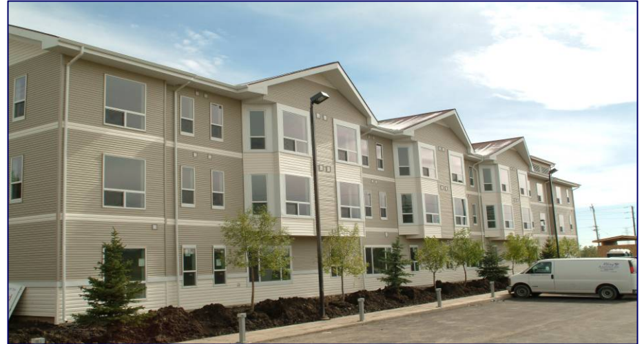
Bob Ward Residence
